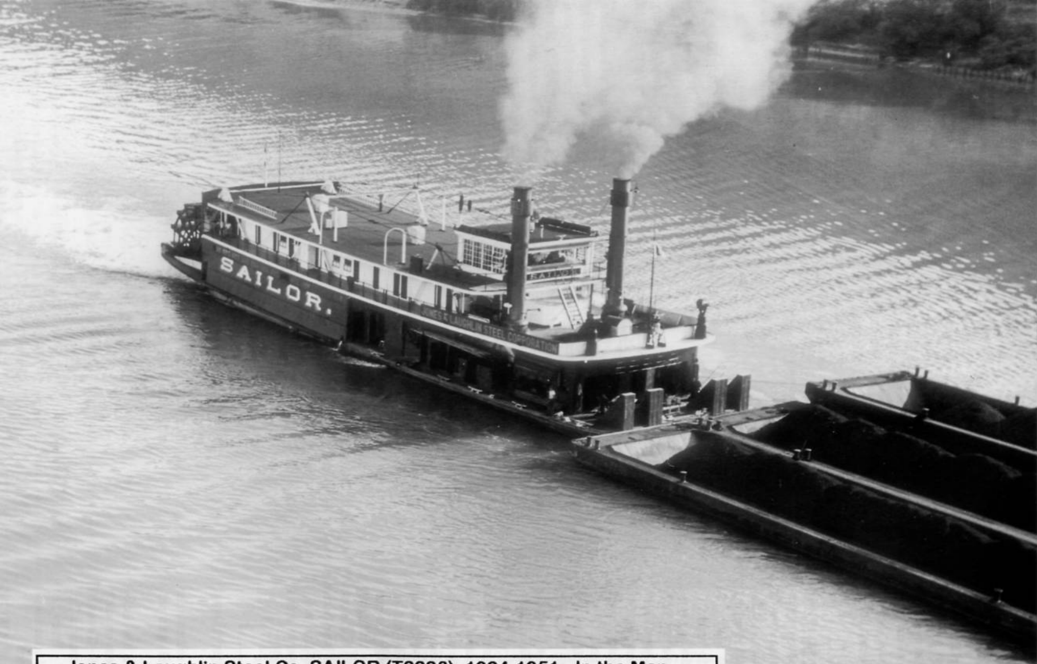
Jones & Laughlin Steel Co. SAILOR (T2226), 1924-1951. In the Mon River pools she was called "The Little Sprague" with the largest engine-room, biggest paddlewheel and most spacious pilothouse.
