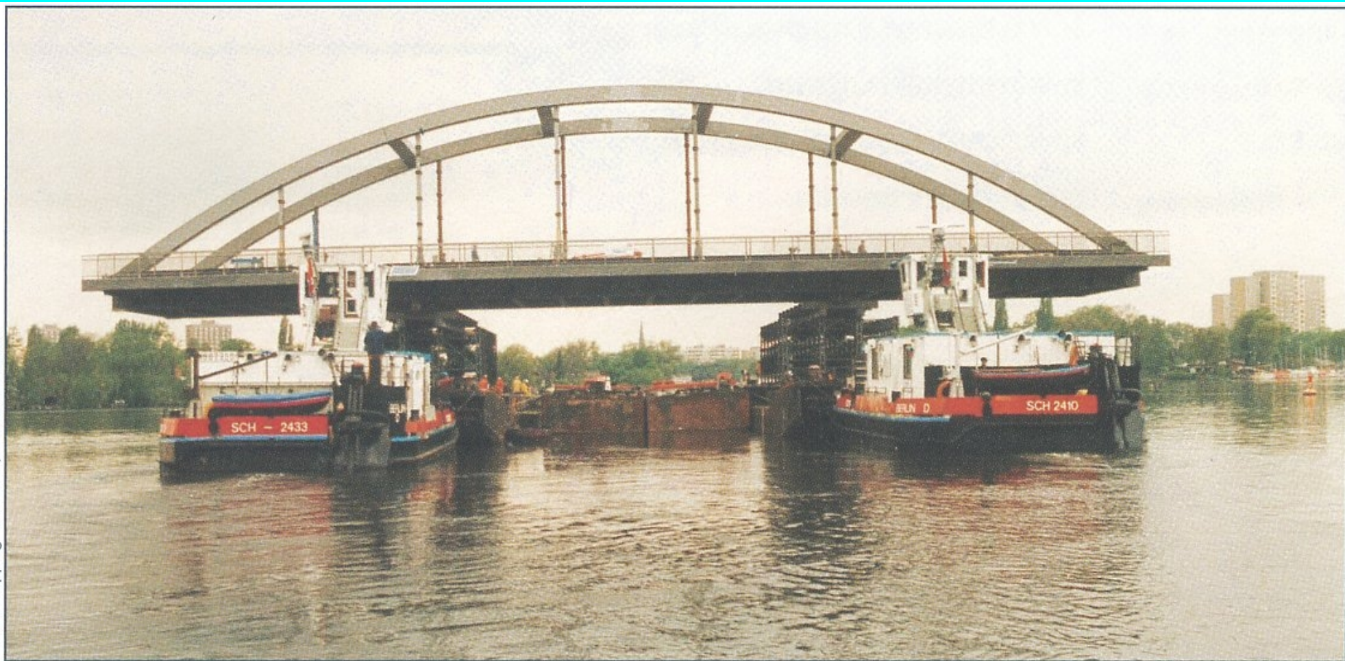
A tandem of two barges transports the center span of a bridge along a waterway in Germany.
