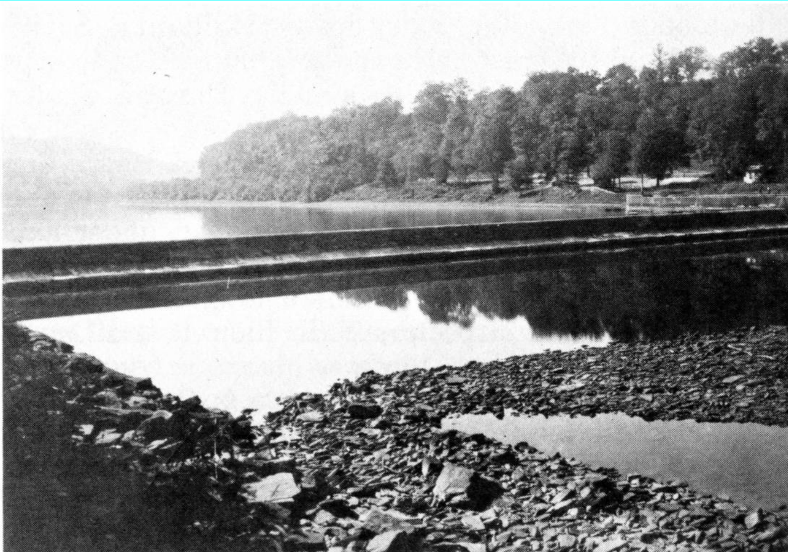
October 2, 1930, Lock & Dam 11, Monongahela River
