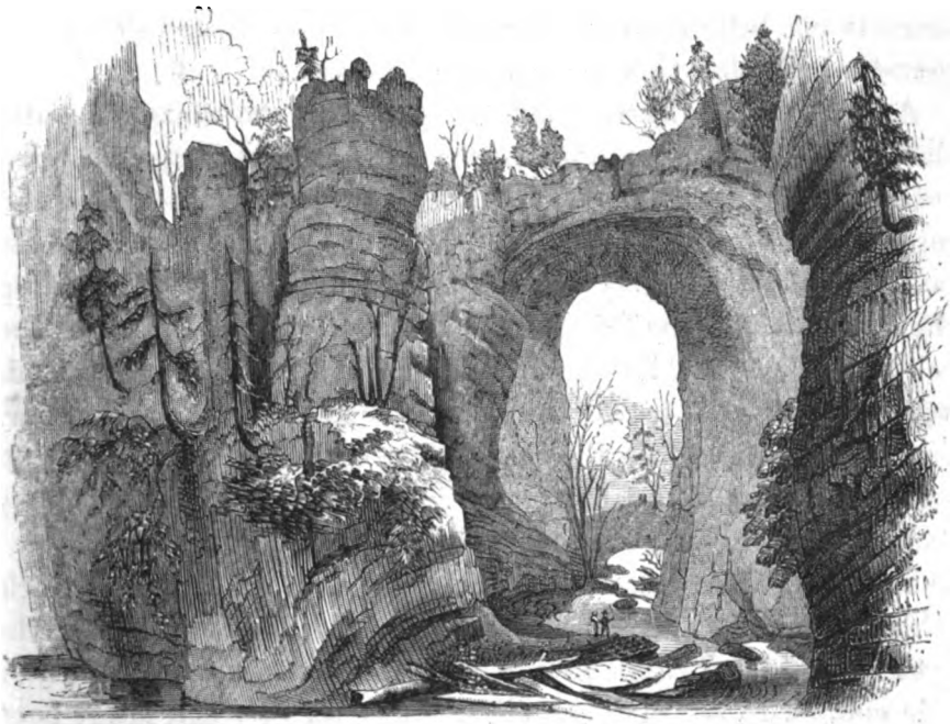
VIEW OF BRIDGE, UPPER SIDE.
