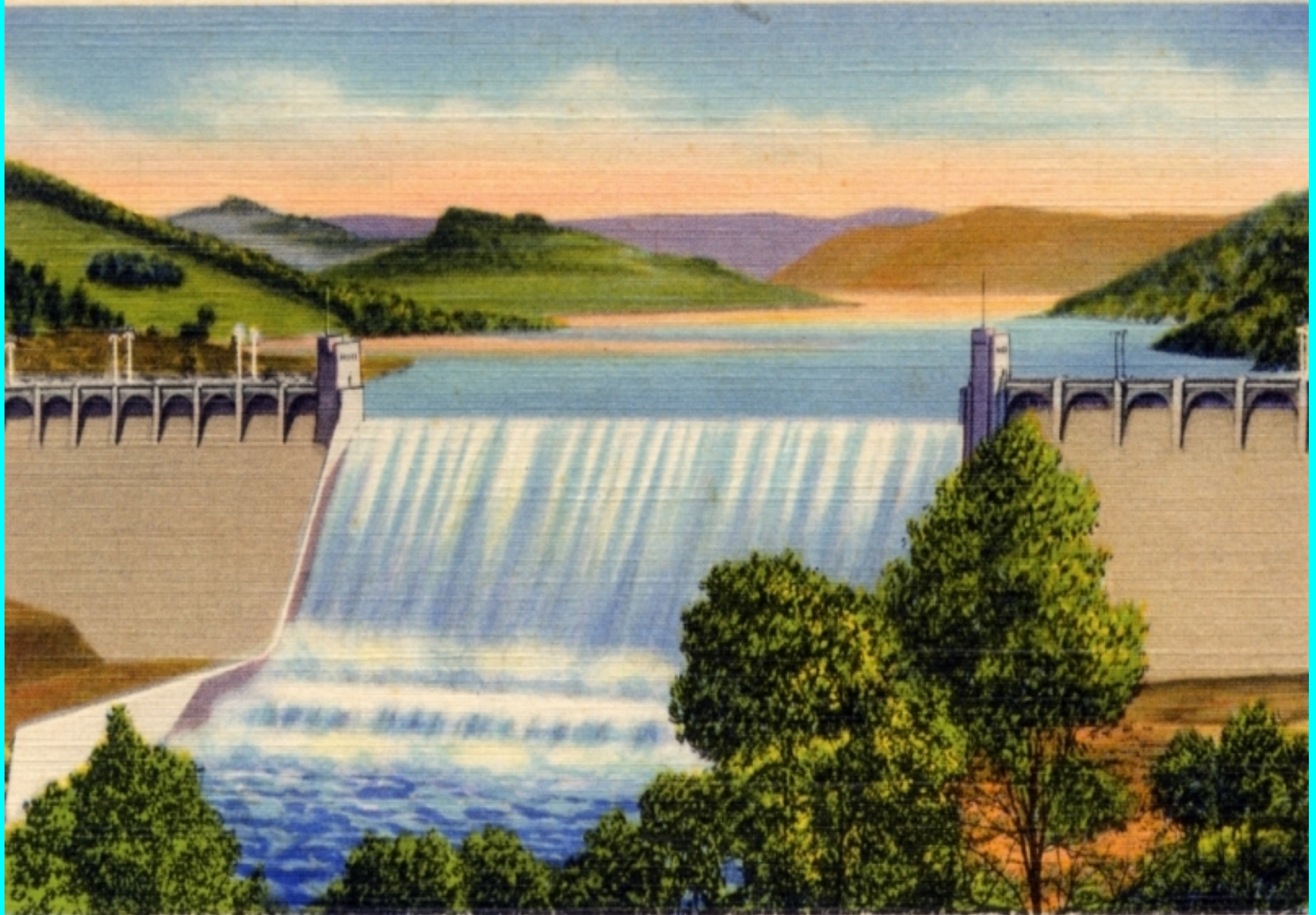
Tygart Valley Flood Control Dam on Tygart River near Grafton and Clarksburg, W. Va.
