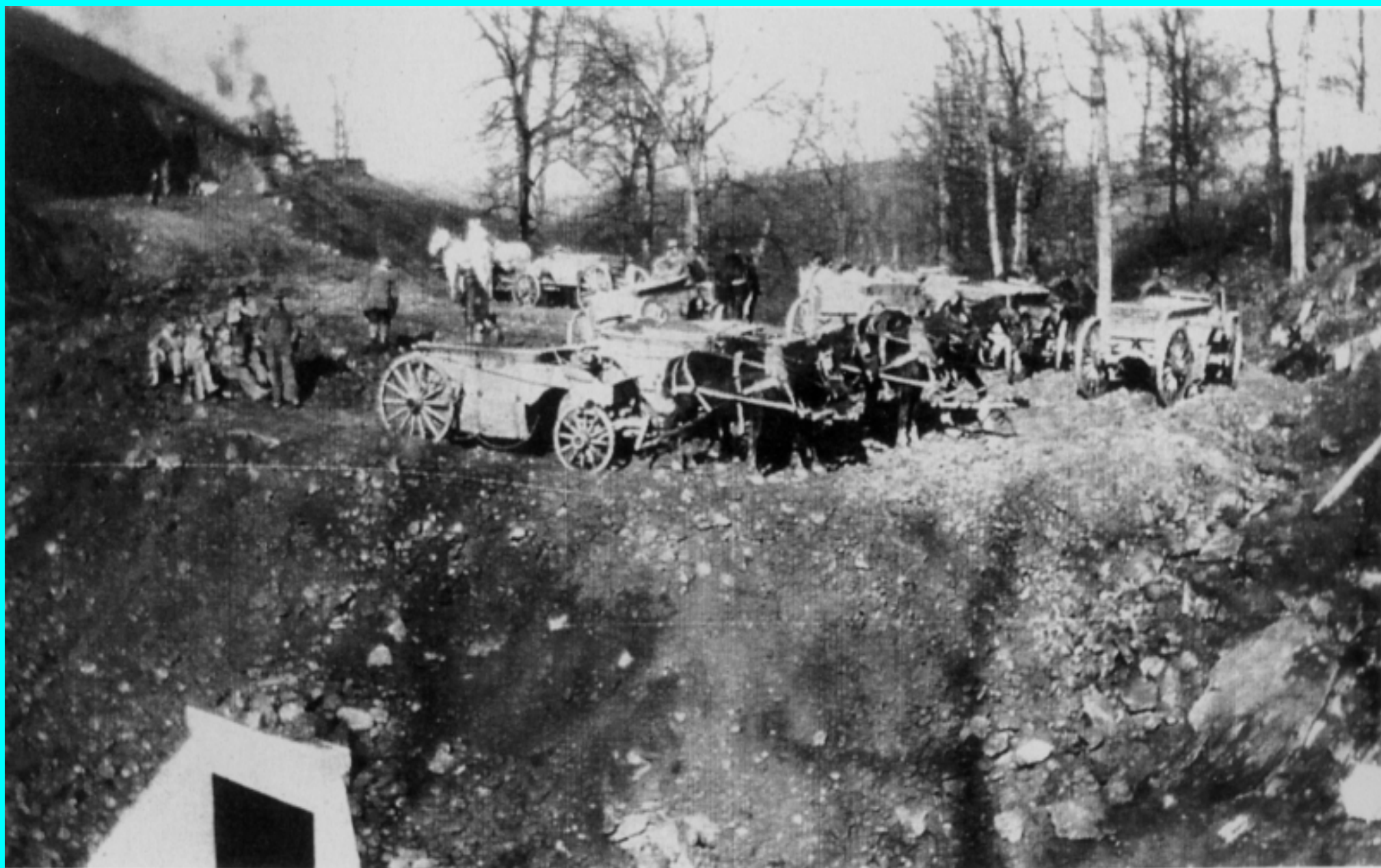
Road building on Route 7, 1929.
