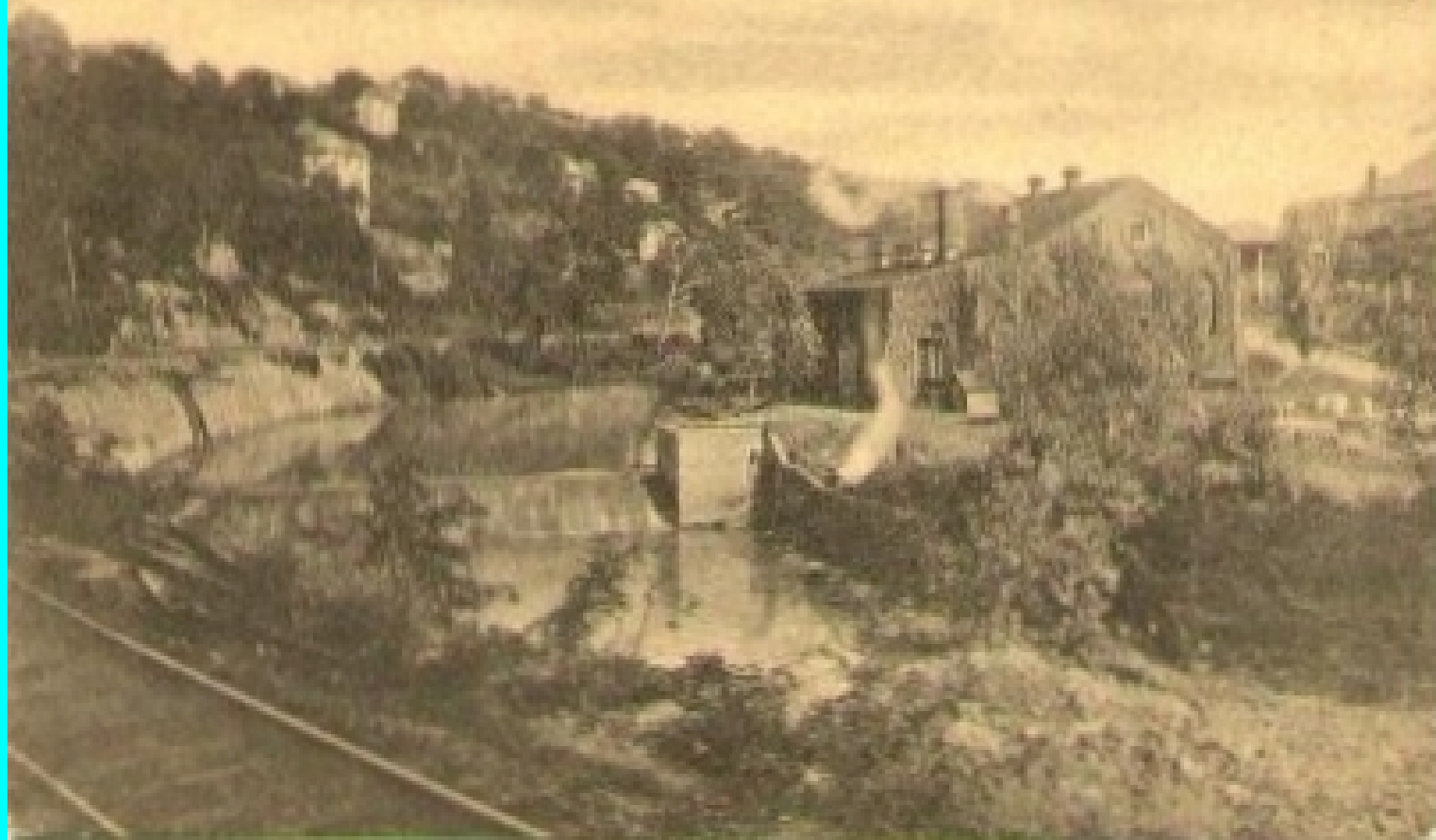
Power House and Dam W. Va. Traction and Power Co., Morgantown, W. Va.
