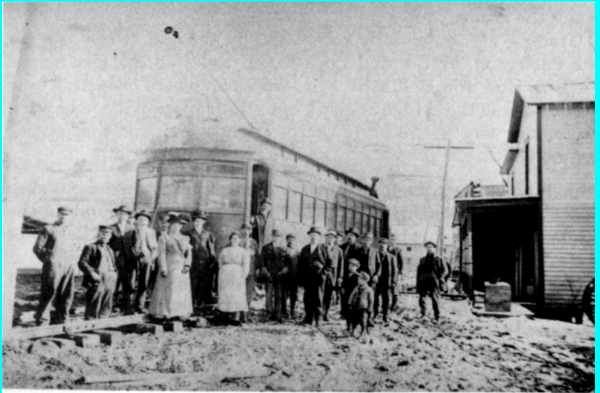
The first M.&D.V. trolley car in front of Ed Goodrich's Store in Osage.
