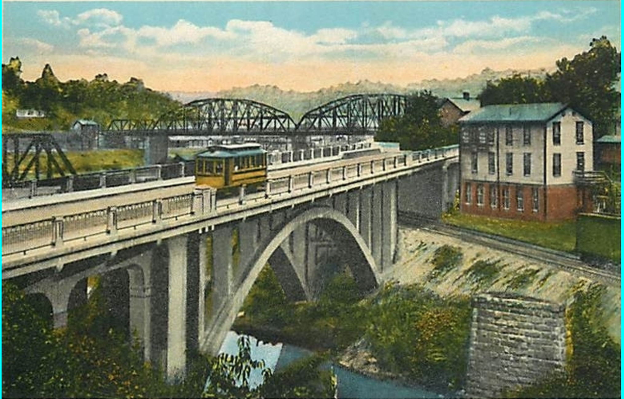
BRIDGE STREET BRIDGE AND PLEASANT STREET BRIDGE, MORGANTOWN, W. VA.
